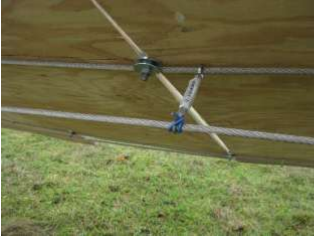
Cross Tie Turnbuckle (initial installation)
