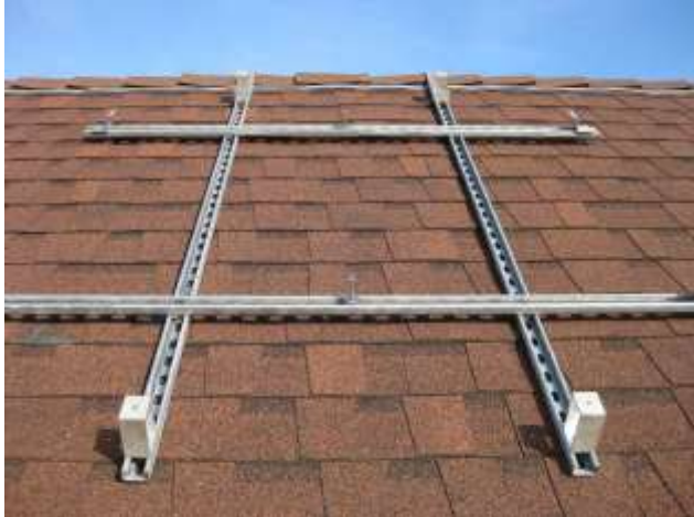
Small rails can be carried up a ladder and placed
