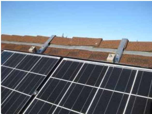
PV Clips hold the PV panel prior to clamping
