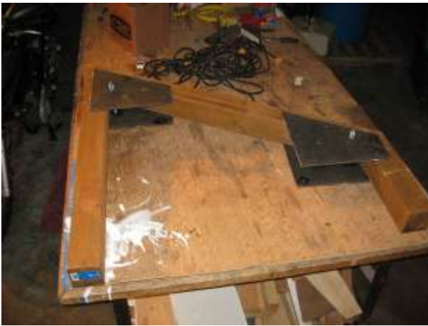
A Cross Brace is added next for front back stability
