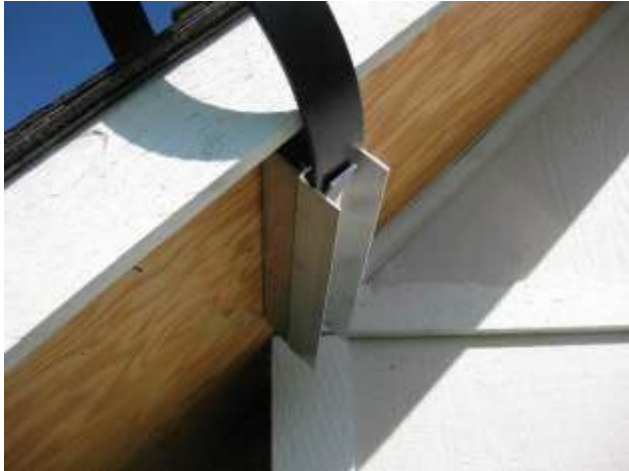
Pivot Joint (initial design prior to universal joint)
