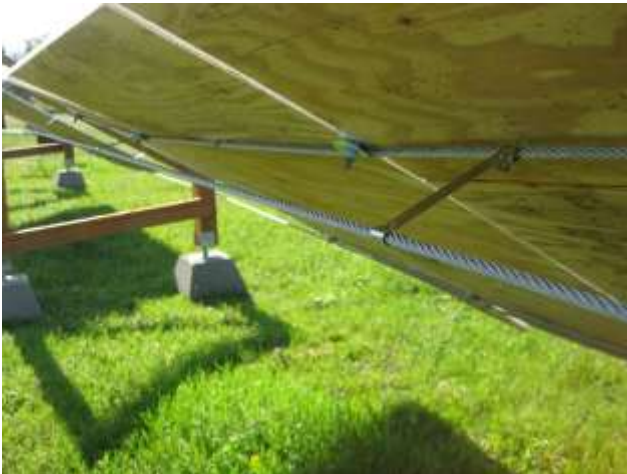
Cross Straps (final installation) held w/ pop rivets
