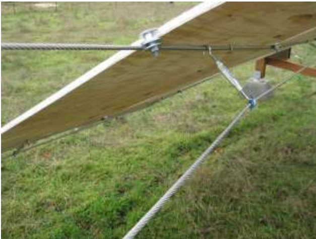
Turnbuckles allow capturing cross tie length
