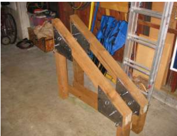
The cut ends still need soaking coats of preservative
