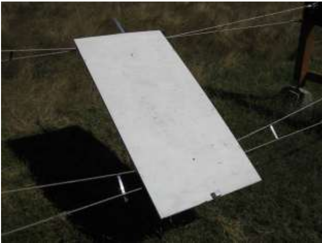
PV Hanger holds PV panel before clamping
