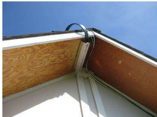
TCS R1 holding real PV panels. [Previous Design]
