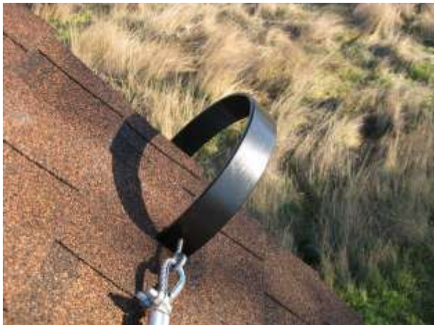
GM Mount w/ Pull Tensioner (Pad not installed yet)
