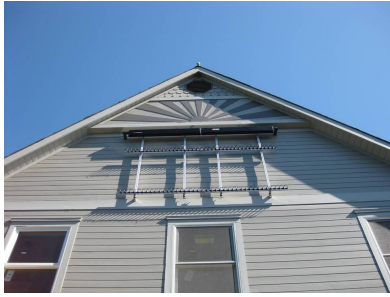
SW Facing Wall (E-Tubes)
