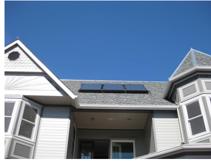
SE Facing Roof (Flat Plate)
