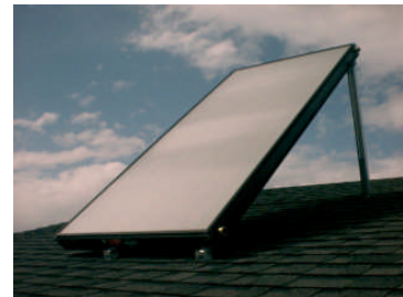
The Gobi 3366 flat plate collector provides a heated glycol and water solution circulated with an adjacent solar energized DC pump. This 4 x 7 collector supplies a preheat system in Sequim.
