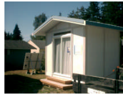
The new main office of Olympic Energy Systems, Inc. is still keeping warm with about 8 KWh per day in Winter, with curtains to keep the summer sun out!
