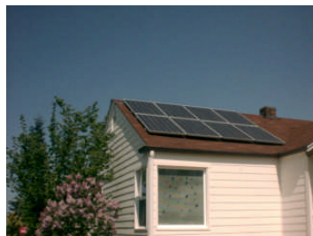
Installation is already underway to put a 3200 Watt PV array on this roof, above and to the east of a 30 evacuated tube solar hot water collector for a preheat system in Sequim.
