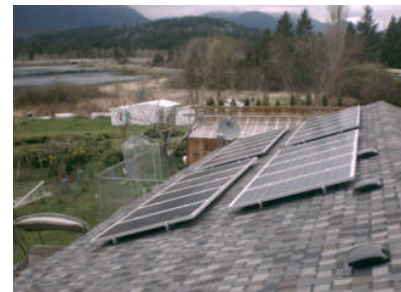
The second phase of this project resulted in an additional 1750 Watts of grid-tied solar energy production, for a total 3500 Watts.
