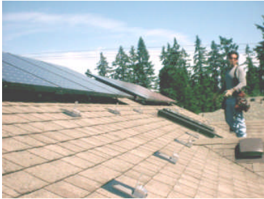
These Sanyo 200 Watt panels in Kirkland are of the highest efficiency (17%) available on the commercial market. There are two parallel strings being added one year after the first set, totaling 4000 Watts.
